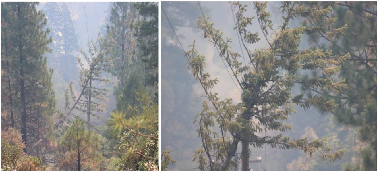
27 Douglas Fir Tree leaning into PG&E’s Lines
